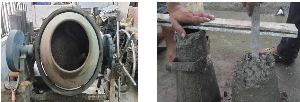
Figure 3.12: Mixing of Concrete
