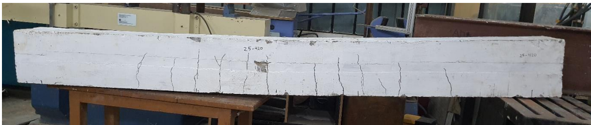
Figure 3.21: Cracks in beam reinforced with B420DWR and cast with 24.1 MPa concrete
