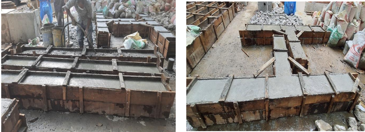
Figure 3.13: Casting of Concrete
