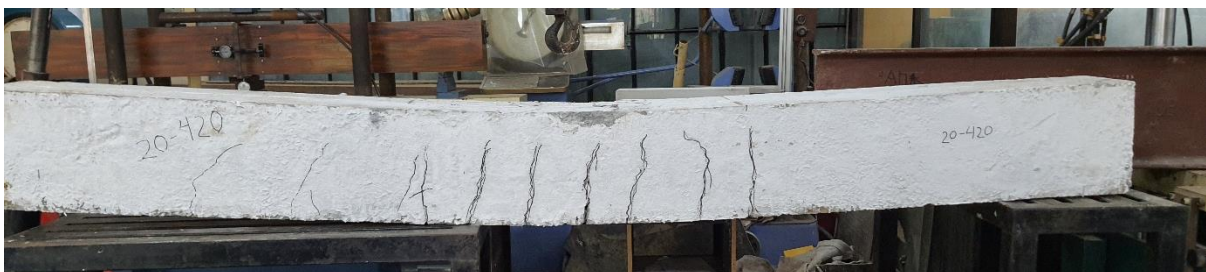
Figure 3.18: Cracks in beam reinforced with B420DWR and cast with 17.2 MPa concrete
