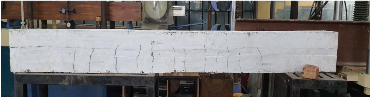
Figure 3.23: Cracks in beam reinforced with B600C-R and cast with 24.1 MPa concrete
