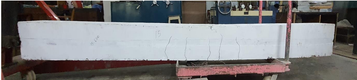
Figure 3.20: Cracks in beam reinforced with B600C-R and cast with 17.2 MPa concrete
