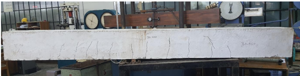
Figure 3.25: Cracks in beam reinforced with B500CWR and cast with 29.3 MPa concrete
