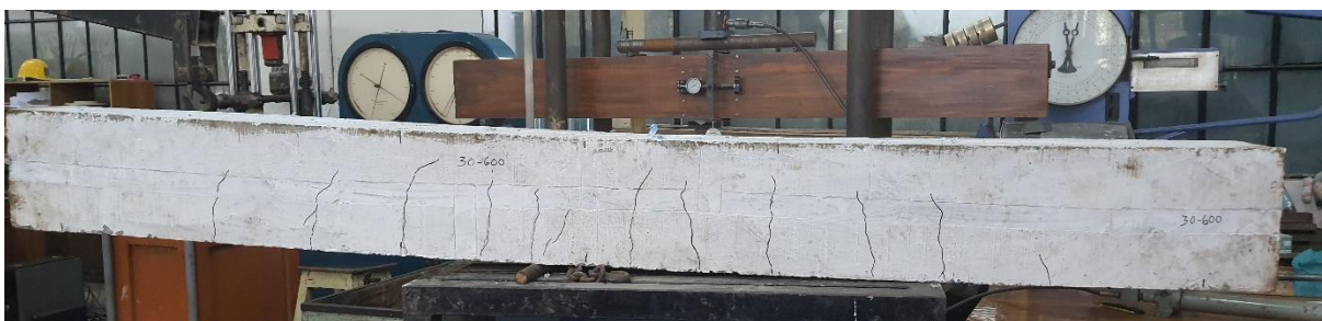
Figure 3.26: Cracks in beam reinforced with B600C-R and cast with 29.3 MPa concrete
