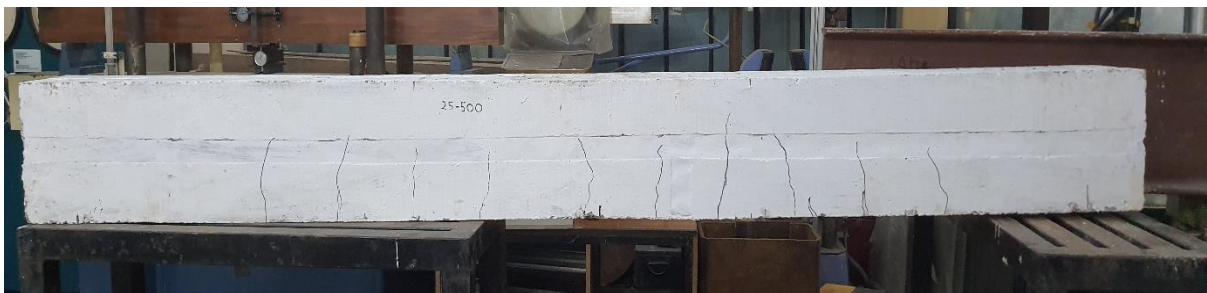
Figure 3.22: Cracks in beam reinforced with B500CWR and cast with 24.1 MPa concrete
