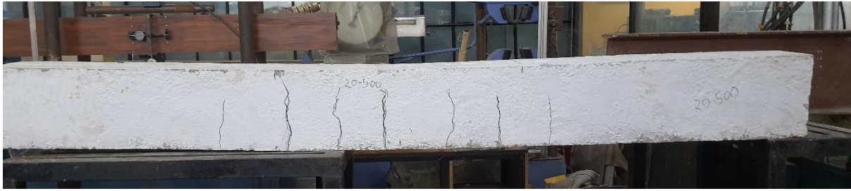
Figure 3.19: Cracks in beam reinforced with B500CWR and cast with 17.2 MPa concrete
