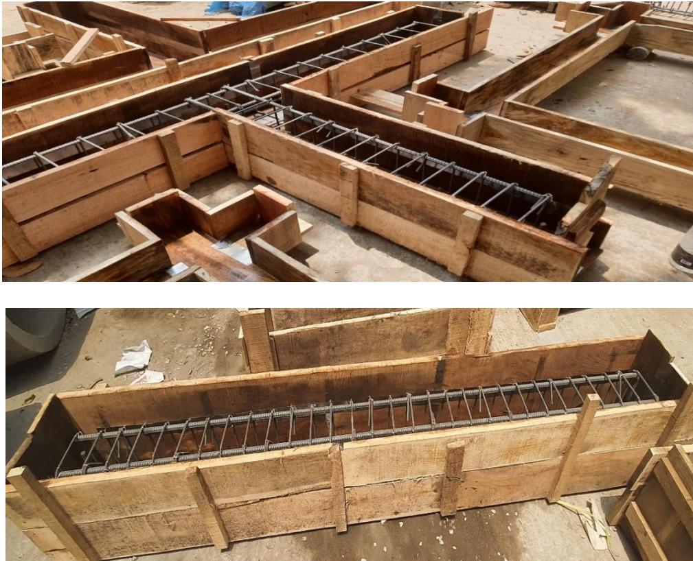
Figure 3.11: Formwork Preparation
