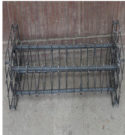
Figure 3.10: Reinforcement Preparation
